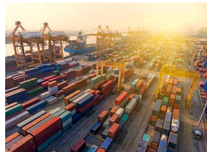
Modern container handling is a logistical challenge.
